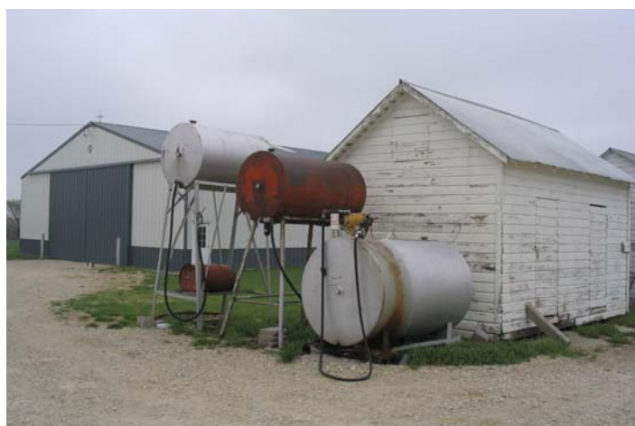
BEFORE: The former fuel storage system on Chris Visser’s farm included a diesel tank with a seep. After completing the RFFP environmental assessment, Chris saw the need to replace the tank and implement containment tanks. Photo by Mary
