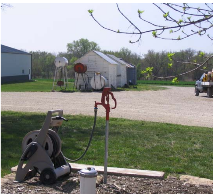
BEFORE: The above photo illustrates the proximity of the leaking fuel storage tanks to the family's drinking water well. This was a major water quality concern. Photo by Mary Howell
