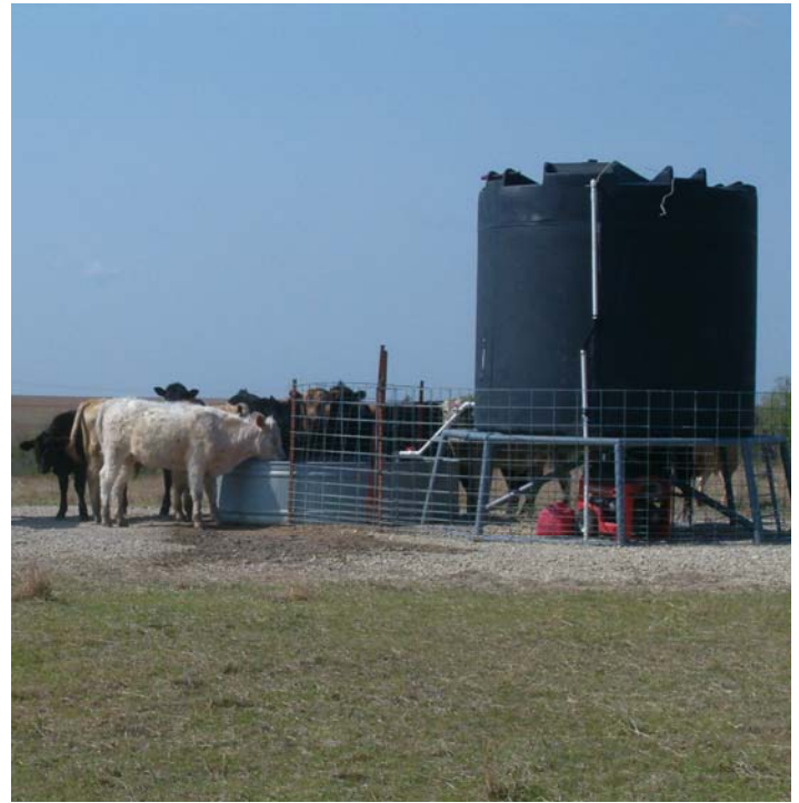
Don Walenta installed a 3,000 gallon storage tank and 500 gallon drinking tank, both supplied by a well on his Butler County ranch. A gas-powered generator powers the pump on the well. Don utilizes a rotational grazing system, therefore the alternative system supplies water to his cattle when they are in that portion of the pasture.
