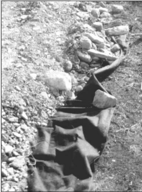
Ken built a couple of stream crossings (right) for his cattle, using gravel over engineering fabric. The fabric (left) will help keep the gravel from sinking into the mud during wet weather, and is cheaper than concrete.
